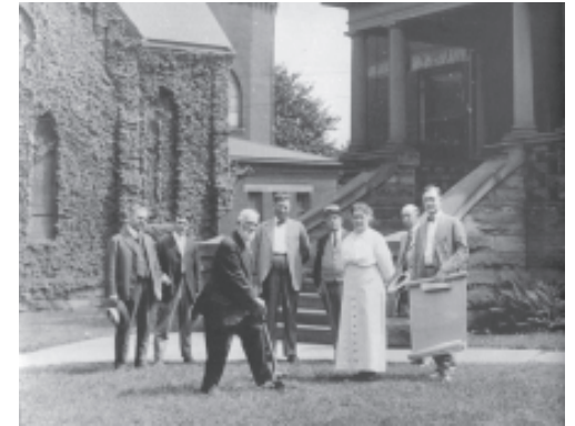
Groundbreaking for the 1901 or 1903 addition to the hospital
